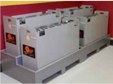
In Progress Install
