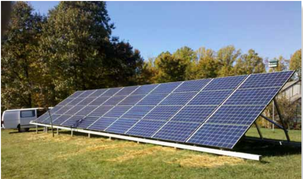
Photo courtesy of Joshua Galante of Altered Energy: Ground mount system.
