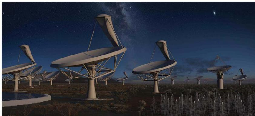
**[FIG1]** An artist's rendition of the SKA dish arrays in operation at night. Using a technique known as interferometry, they will be able to combine their data to create an image that would be the same as one created by a much larger single aperture instrument. (Photo courtesy of the SKA Organisation.)
